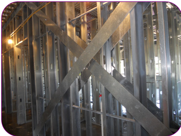
Fig 5. Detail of Shear wall X- Bracing
